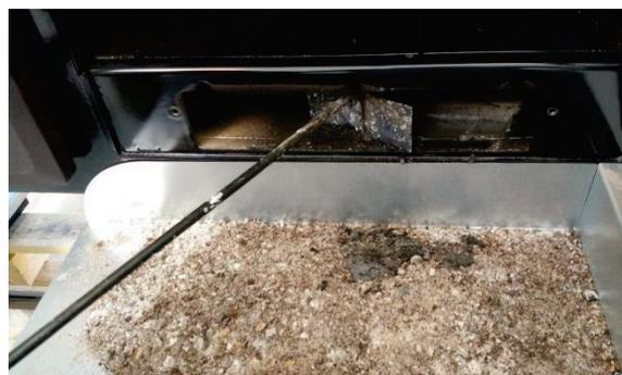
*Figure No.18 - Accesses via which to clean the flue socket.*
